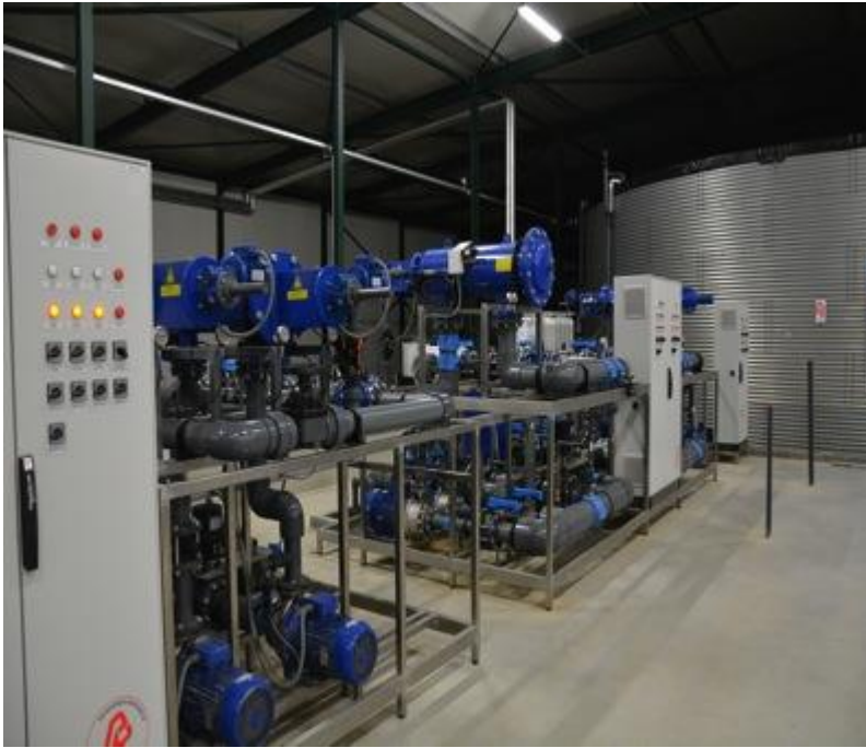
Figure 8. Fertigation equipment for a 10 hectare tomato nursery (Holland, 2014)
