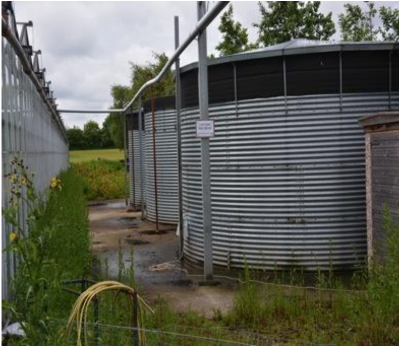
Figure 10. Slow sand filtration tanks on a tomato nursery using drainwater recirculation (UK, 2014)
